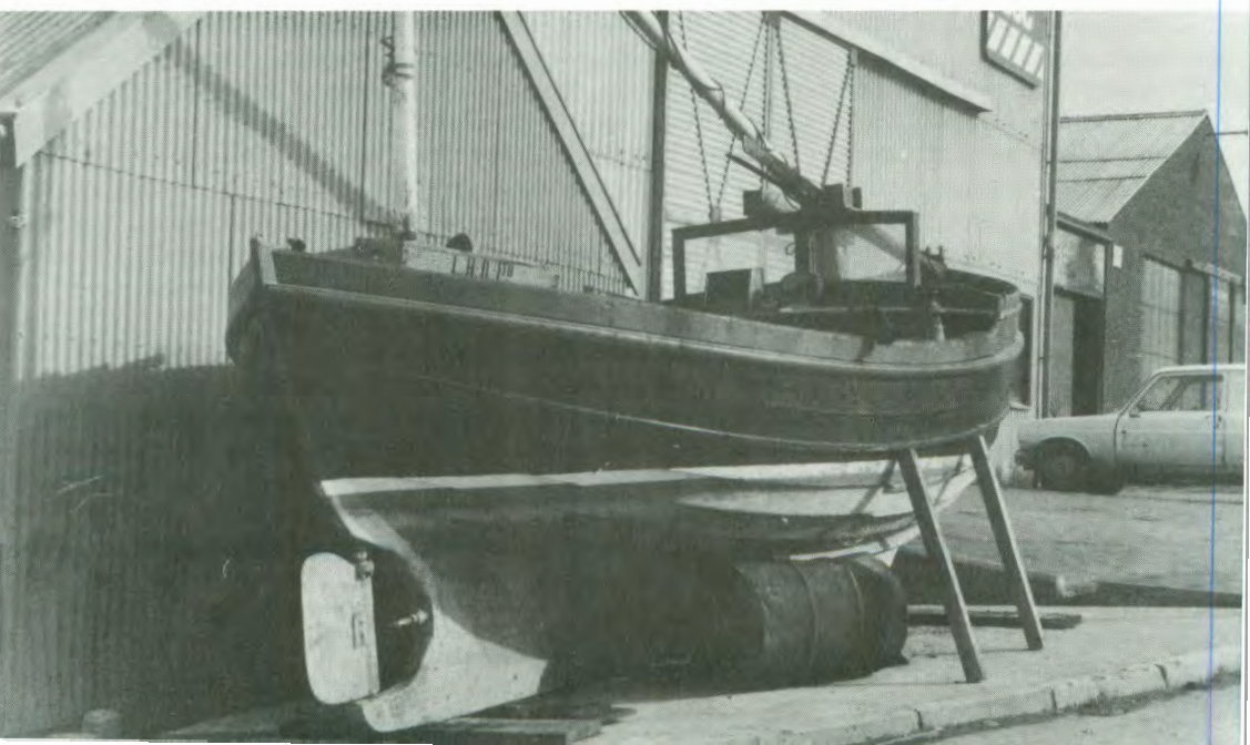
Figs. 8.3; 8.4.— Bow and stern three-quarter views of the UTILISE, LK 589. This is a fine example of the purpose-built motor craft built by Walter and Phillip Duncan for the inshore fishery during recent years. The lines of hull and planking, the functionalism of layout and fittings, epitomise attitudes and skills that represent the best of the ongoing Scandinavian tradition in Shetland. (Photographs: A.G. Osler)
