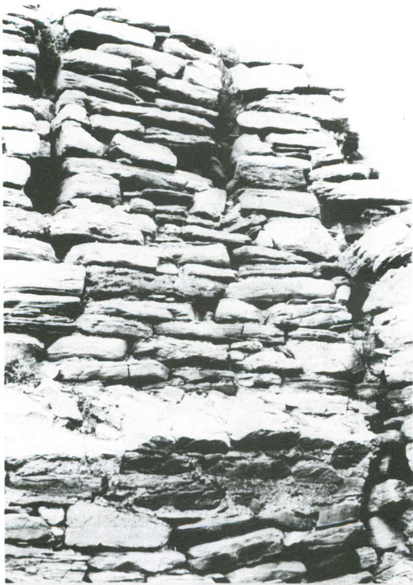
Fig. 3. Inside of upper structure, Caisteal Bharraich, showing a combination of possible attic beam holes and slots for roofing couples, suggesting a possible lowering of the roof. The abutment on the lower edge may have been corbelling or support for an upper floor. (Photo: Dr Joanna Close-Brooks, 1985)
