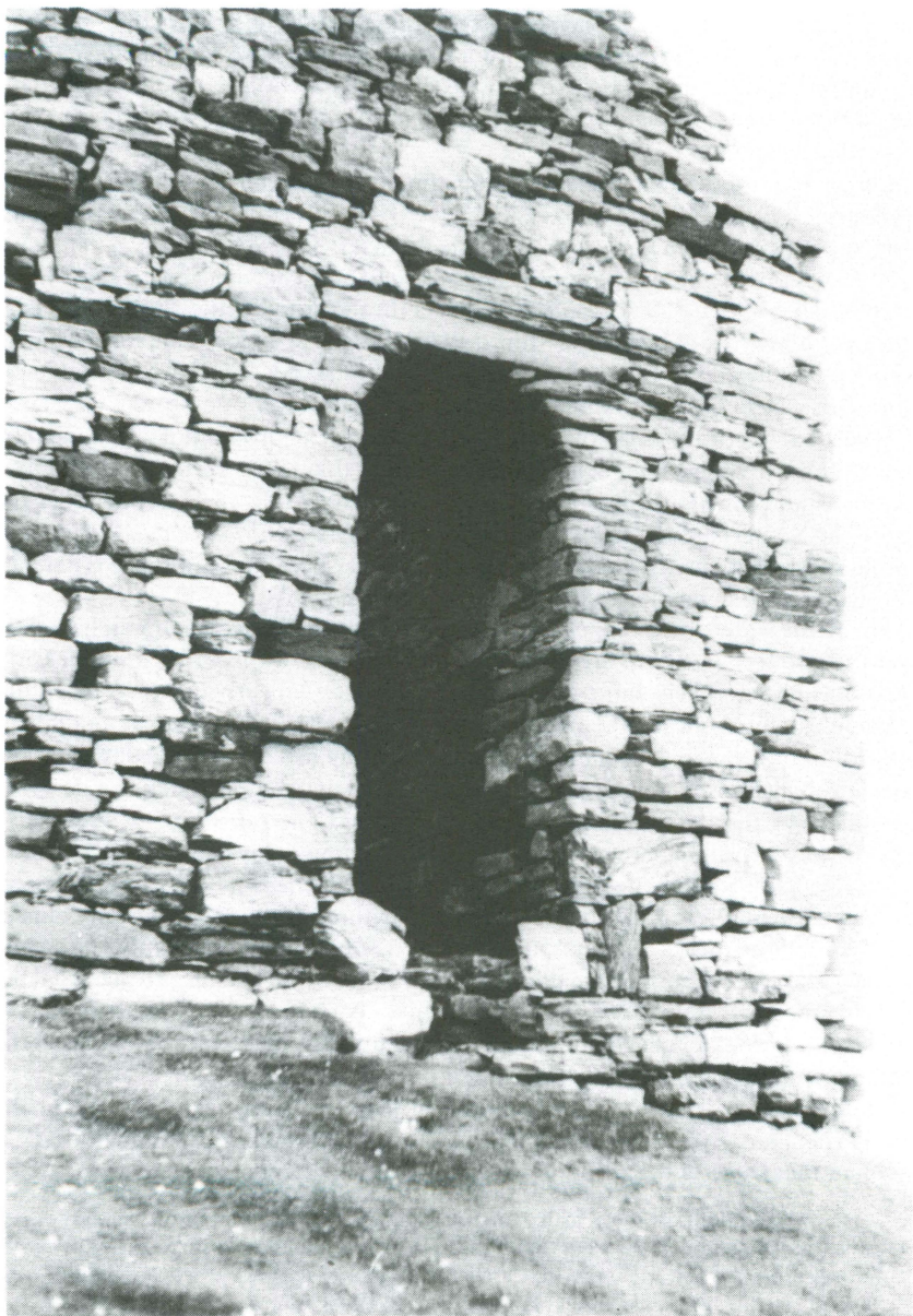
Fig. 2. Doorway, Caisteal Bharraich, showing the character of the masonry; the aperture shows signs of possible rebuilding. (Photo: Dr Joanna Close-Brooks, 1985)
