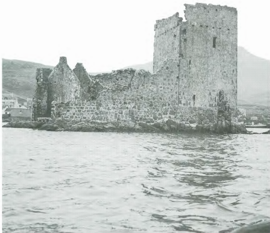
Figure 3. Kisimul Castle in 1956: exterior from south, showing joint between tower and curtain wall. The gap in the curtain wall to the left is where the Tanist House now stands. The gables beyond belong to the hall and its addition. Crown copyright reproduced courtesy of Historic Scotland.
