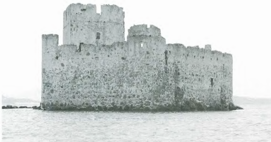
Figure 4. Kisimul Castle in 1956: exterior from the northeast. The wall to the right of the prison tower shows evidence for heightening of the wall, details now largely lost under concrete render. Crown copyright reproduced courtesy of Historic Scotland.
