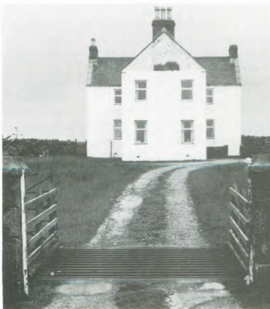
Fig. 6.6 Free Church of Scotland, Achiltibuie, 1992. The slate roof was replaced with blue corrugated asbestos ca. 1990, when other repairs were made.
