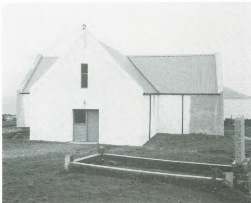
Fig. 6.6 Free Church of Scotland, Achiltibuie, 1992. The slate roof was replaced with blue corrugated asbestos ca. 1990, when other repairs were made.
