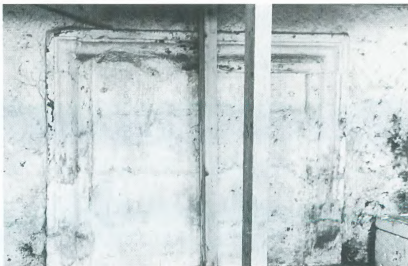
Fig. 7.22 Garden pavilion: blocked hearth in ground floor with bolection moulded surround. 1994.
