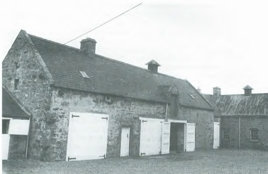
Fig. 7.25 Bighouse: ?former kiln-barn; note vent immediately below eaves and another in gable end. 1994.
