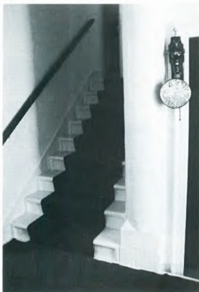
Fig. 7.13 Bighouse Lodge: stone scale and platt staircase. Note centre spine wall rounded at landing face, with square base and capital. Also moulded risers to stone stairs. 1982.
