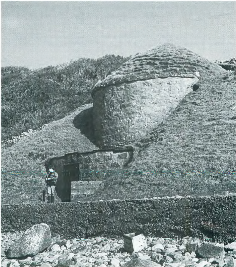
Fig. 7.28 Icehouse. Bowed ante-chamber fronts lower portion: chute to rear of turf conical roof. 1992.
