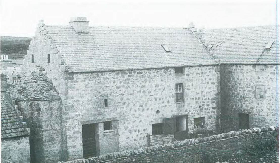
Fig. 7.26 Sandside, kiln-barn: the kiln occupied the left hand section, the upper floor reached by staircase in canted stairwell fronting gable end. 1992.
