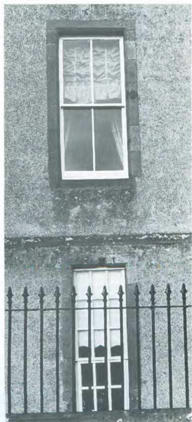
Fig. 7.12 Bighouse Lodge: narrow raised basement window with scarcement (ledge) and wider window above, 1994.
