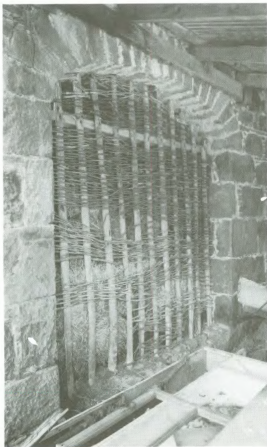
Fig. 8.37 Wattled ventilation panel in east wall of heather-thatched barn. Mains Farm, Applecross, ca. 1976.
