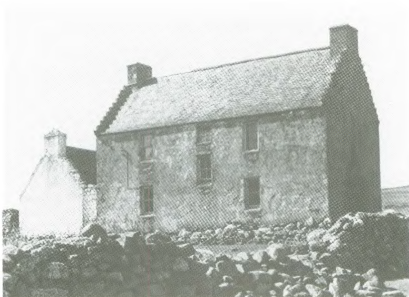
Fig. 8.20 Udrigle, 1745. South front: note off-set centre windows lighting half landings. 1955.
