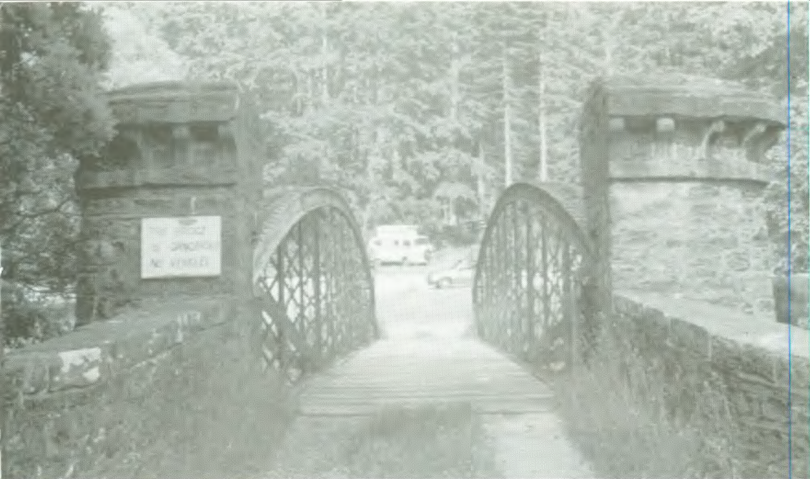
Fig. 8.34 Auchindrean Bridge, designed ca. 1870 by Sir John Fowler of Braemore: rare lenticular (fish eye) truss bridge with masonry end piers. 1989.
