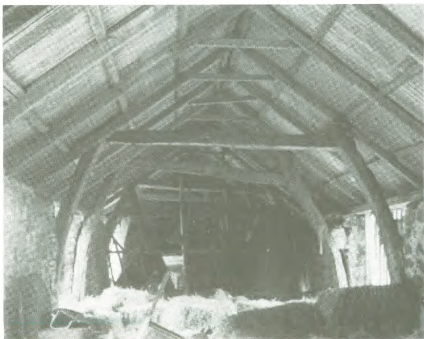
Fig. 8.35 Kerrysdale: interior of cruck-framed barn. Cruck blades have been sawn off above tie-beams to accommodate shallower pitch of replacement corrugated-iron roof. 1981.
