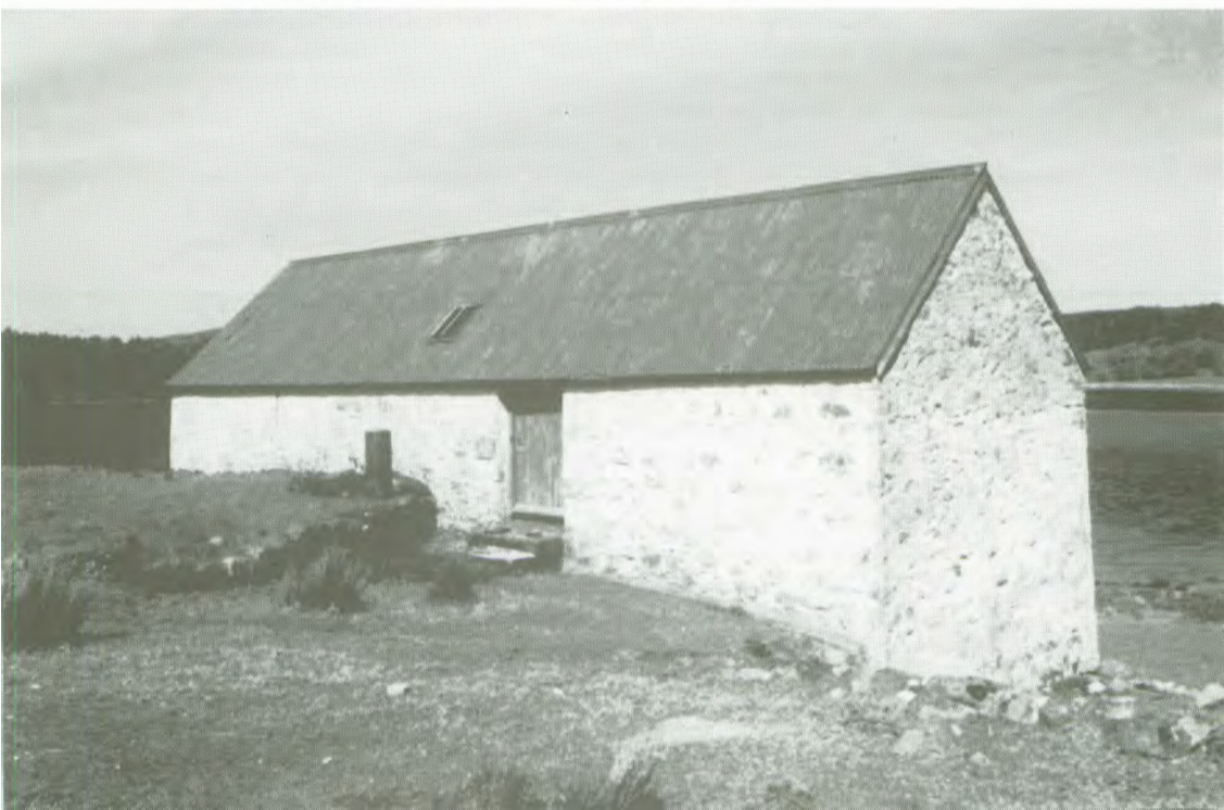
Fig. 8.39 Bank barn, Poolewe — rear elevation, showing direct access from slope to upper floor and a horse-gang to the left of the (west) doorway. 1989.
