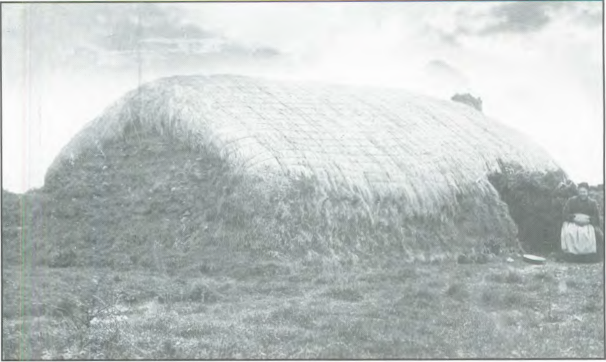
Figure 5: Mrs Mary Gilrea's sod cottage in the parish of Jurby, c1897; she was known as 'Gilrea of the Gorse'. The walls were built entirely of sod blocks and the roof was thatched with Marram grass.
