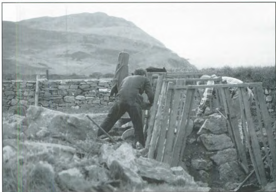
Figure 3: A stone-faced hedge being constructed at Manx National Heritage's farm at Cregneash in 1997. This was part of a competition designed to help preserve such skills.
