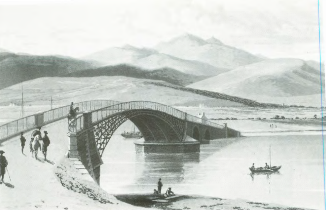
Fig. 12.22 The iron Telford bridge at Bonar had a 150 ft (45.7 m) main span. William Daniell aquatint, 1821.
