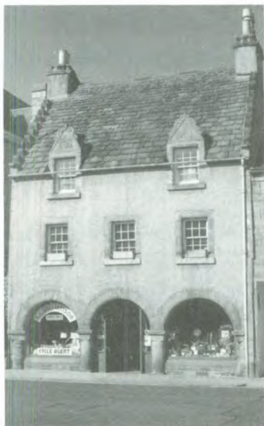
Fig.12.3 Braco's Banking House, Elgin, 1694. Harled rubble, tooled and polished sandstone ashlar dressings; sandstone slab roof.
