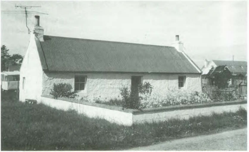
Fig.12.9 16 Bogmuir, near Fochabers, 1828. 'Clay and bool' cottage; note horizontal lines indicating the courses, each of which was allowed to dry out before the next addition. Corrugated iron roof replaces former 'clay' thatch. (Crown Copyright: Historic Scotland)
