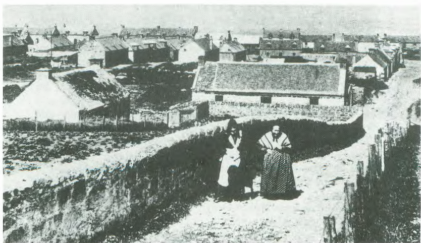
Fig.12.11 Hopeman, circa 1900. Clay thatched cottages; the centre cottage is in process of being re-thatched and the underlay of divots is clearly visible. Note clay slurry on roof of left hand cottage.
