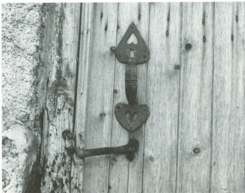
Fig.12.19 Easter Claggan, Inveravon. Blacksmith crafted iron door handle (probably late 18th or early 19th century).
