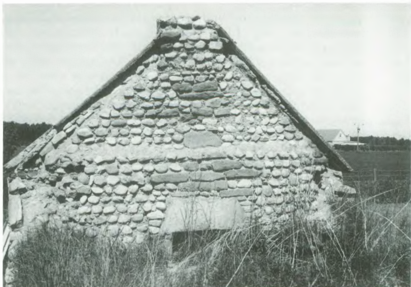
Fig.12.10 Cowfurach, near Broadley. 'Clay and bool' revealed. (Crown Copyright: Historic Scotland)
