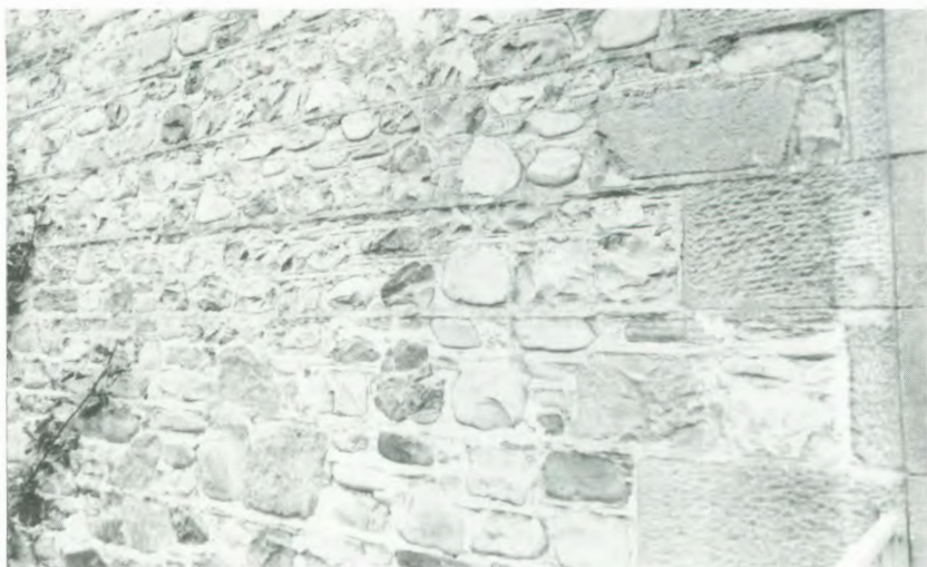
Fig.12.7 2 East Street, Fochabers. Random rubble laid in courses developed from local clay building technique.
