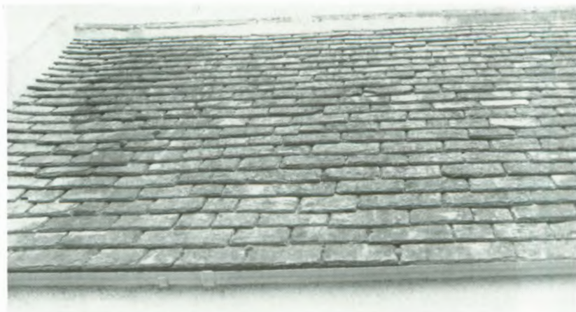
Fig.12.17 Fochabers. Slates from Tarrymount quarries laid in diminishing courses.
