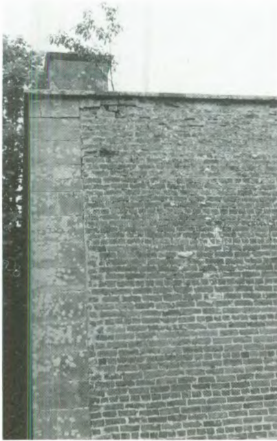
Fig.12.13 Cullen House walled garden, 1788. Brick with Moray sandstone dressings and wallhead chimney stack (some stacks served glass-house and mural heating ducts, some were ornamental). (Crown Copyright: Historic Scotland)
