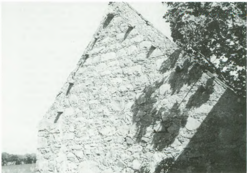
Fig.12.12 Implement shed, Rannas, near Buckie, 18th century. Projecting stone 'pegs' for retaining thatch. (Crown Copyright: Historic Scotland)
