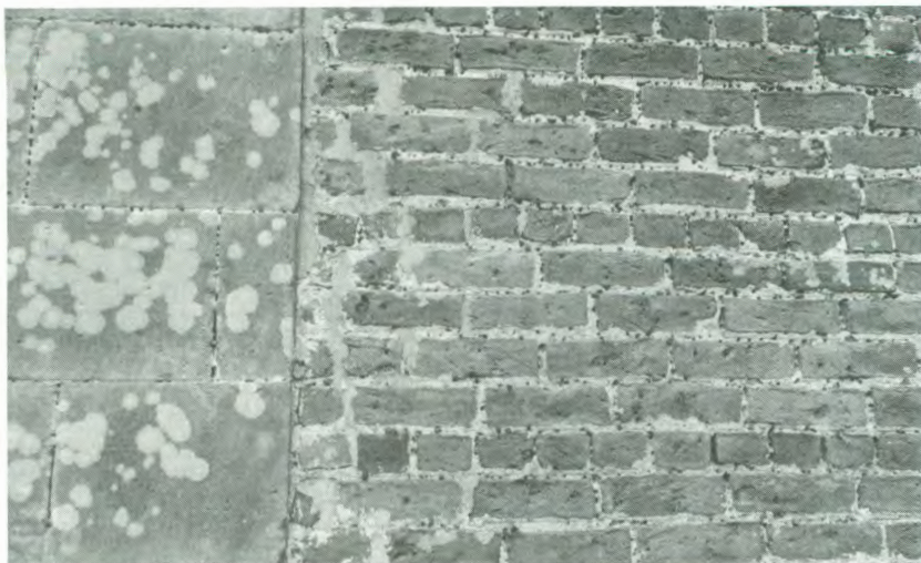
Fig.12.14 Cullen House walled garden, 1788. Detail of close jointed ashlar; also bricks laid in 'English garden bond', 4 rows of 'stretchers' alternated with 1 row of 'headers'. (Crown Copyright: Historic Scotland)
