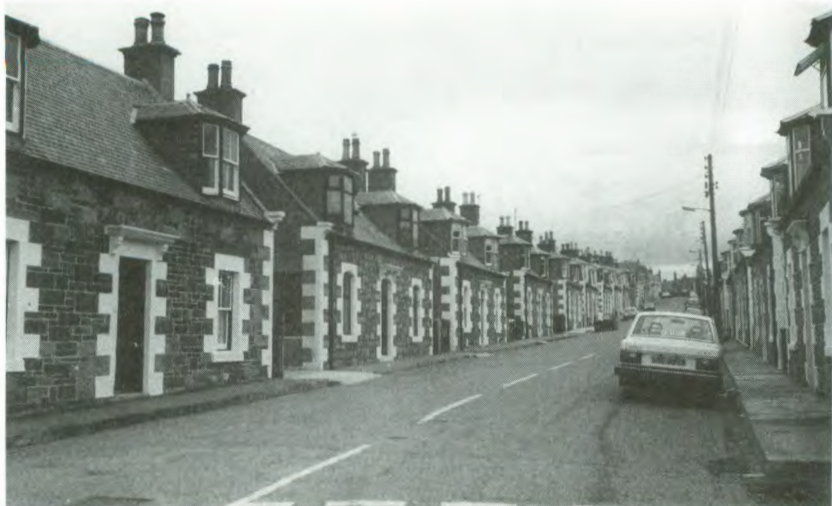
Fig.12.16 Seafield Street, Portknockie, circa 1900. Rubble walling with painted concrete angle and window dressings, cornices and lintels; also flared concrete chimney copes. (Crown Copyright: Historic Scotland)
