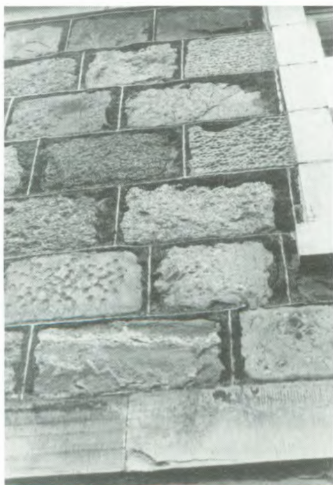
Fig.12.7 2 East Street, Fochabers. Random rubble laid in courses developed from local clay building technique.
