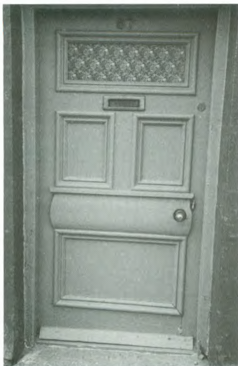
Fig.12.18 Buckie. Banffshire seatown panelled front door with characteristic convex centre rail. (Crown Copyright: Historic Scotland)
