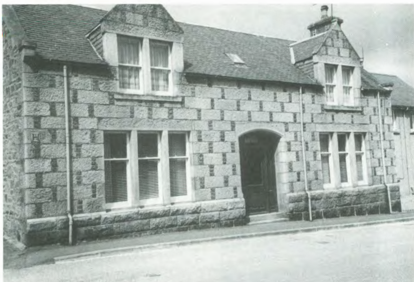
Fig.12.4 124 Land Street, Keith, circa 1900. 'Aberdeen Bonding'; pale grey granite pinned with dark whinstone wedges. (Crown Copyright: Historic Scotland)
