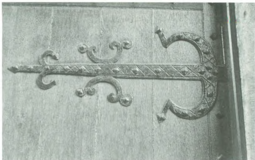
Fig.12.20 South Lodge, Ballindalloch Castle, 1850. Ornate wrought-iron door hinge. (Crown Copyright: Historic Scotland)
