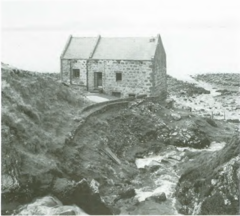
Fig. 14.42 The Estate mill, built ca. 1880. It was obsolete by the beginning of the 20th century, largely on account of the expansion of the railways. Part of the lade survives in the foreground. It led to an overshot wheel. 1992.
