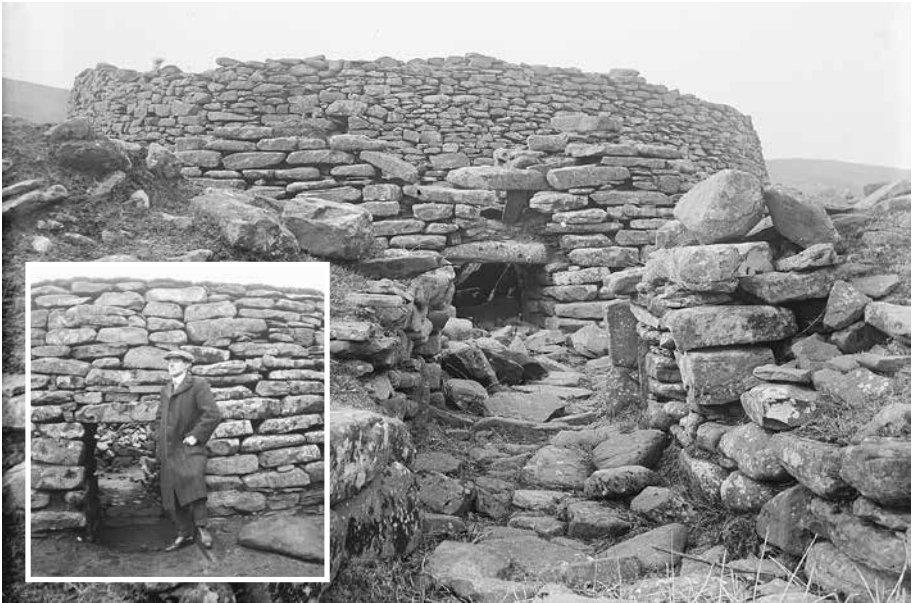
Figures 6-7. Photographs of the forework, c.1906 and c.1908, showing the dereliction and rebuilding. The figure is probably Henry Macleod (1880-1940), clerk of works. Photograph: RCAHMS
