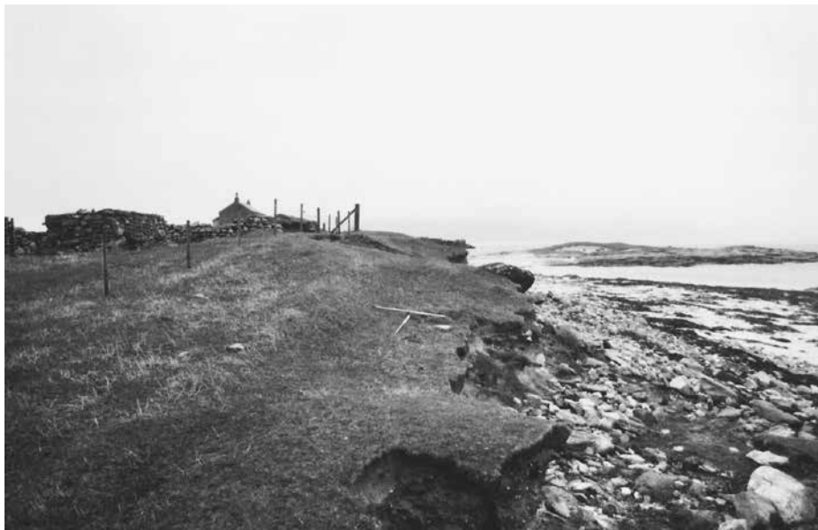
Figure 5: View of St Taran's Chapel under threat of coastal erosion.
